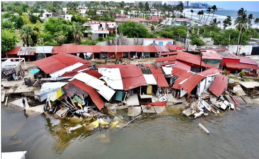
Figure 2. Flooding and destruction of roofs in Guerrero.
